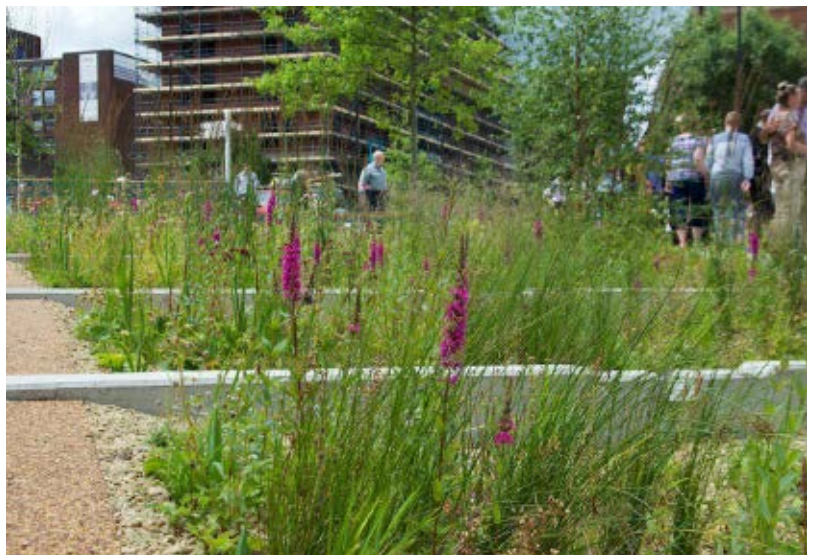
Raingarden and swale
